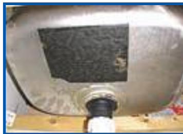
Chrysotile-containing bitumen pad to underside of sink
