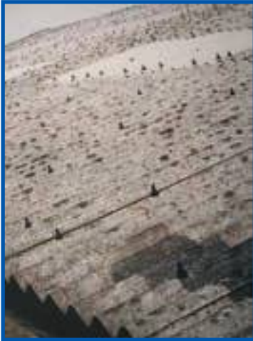
Asbestos cement corrugated roofing
