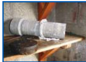
Chrysotile rope to asbestos cement flue pipe
