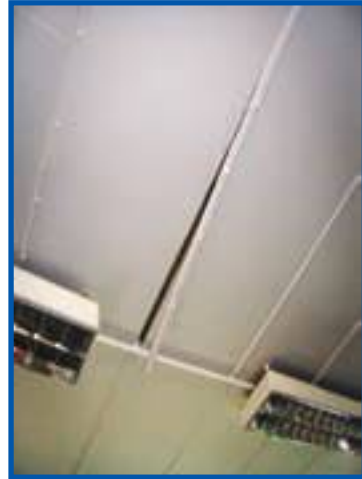
Asbestos cement ceiling panels
