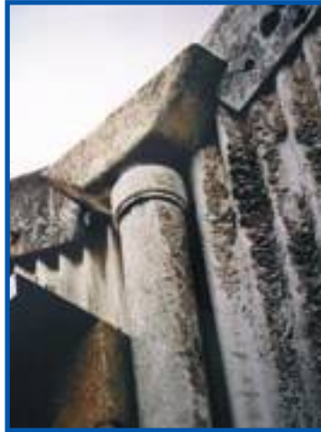
Asbestos cement barge boards and downpipe
