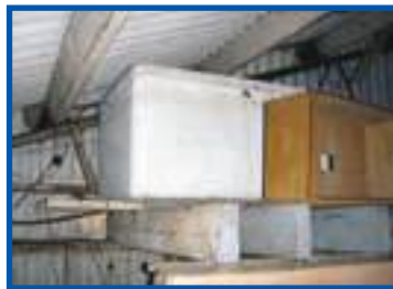
Asbestos cement water tank in attic
