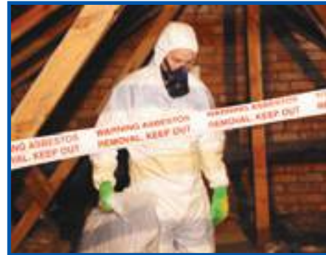
Asbestos worker using orinasal respirator (half mask)
