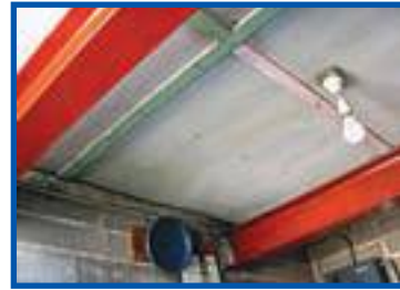
AIB ceiling panels in lift motor room
