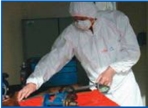
Use of tape and polythene sheeting to protect a work area before cleaning asbestos gaskets from a valve
