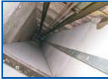
AIB lining to dumb waiter shaft
