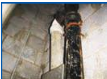
Asbestos cement flue pipe
