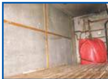
Asbestos cement wall panels in hot press
