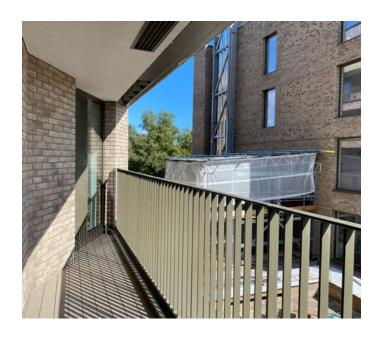
The balconies and facade elements had to be seamlessly integrated with both the brickwork and precast concrete cladding, requiring high levels of precision during both the design and installation phases.
