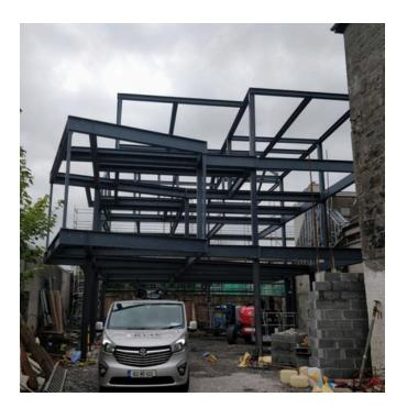
The results demonstrated the effectiveness of the bolted composite system in real-world application. Post-installation inspections confirmed that the beams behaved as unified elements with no observable misalignment, deformation, or slippage.
