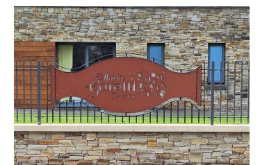
It was constructed with two runs of 50x10 flat bar held apart by 20mm square bars, with the main plate made from 6mm aluminium, copper powder coated, and backed with polished stainless steel. A 40mm void housed LED strips for night-time illumination.
