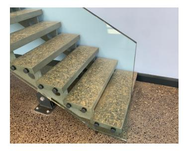
A key fabrication detail involved 3 mm folded stainless steel trays for the concrete treads, with tabs protruding from the main stringers into corresponding slots, allowing for "secret welding" to conceal the fixings.
