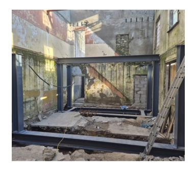
Internally, steelwork was integrated with new concrete slabs and retained masonry, requiring high-precision collaboration with blockwork and follow-on trades. Each phase was sequenced with floor, insulation, and waterproofing works.
