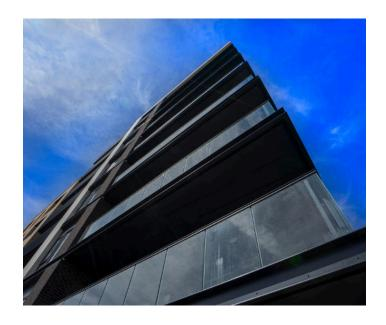
Schöck Isokorb anchors were used for structural support with minimal tolerance.
